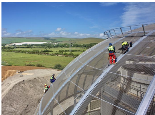
Energy Recovery Facility in Newhaven
